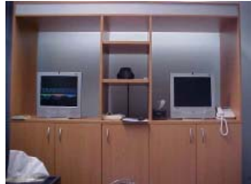
Figure 1b: CCTV room
